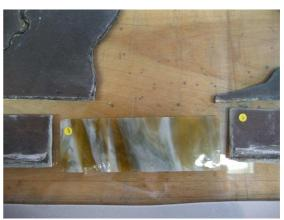
There is a large amount of soot between the layers of glass which could have come from a fire across the street from the church and/or the burning of candles inside the church.
