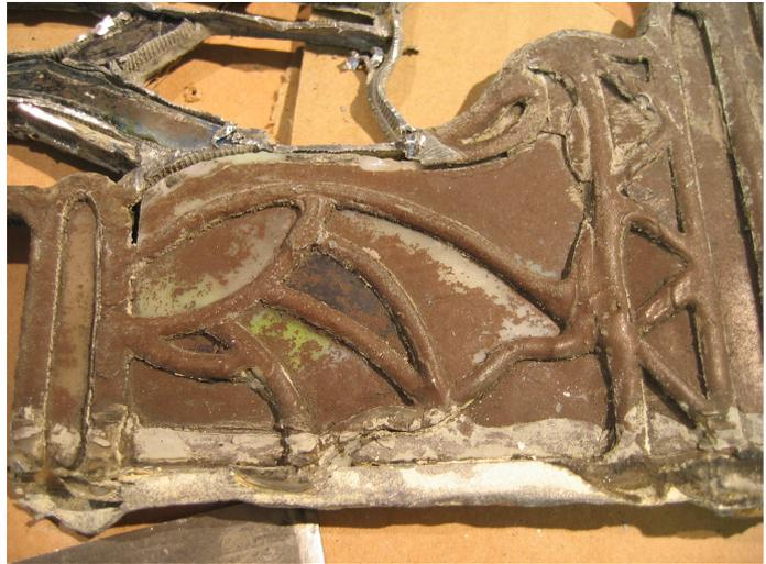
To remove the brown paint, a detergent made of cellulose “Safest Stripper” (3M / Dimethyl adipate, Dimethyl glutarate), harmless for the glass, is very convenient because it can be laid on the glass as a gel. The pieces are soaked half an hour and then rinsed under water.
